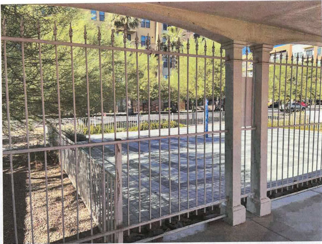
Figure 7: Southside Fencing _ II
